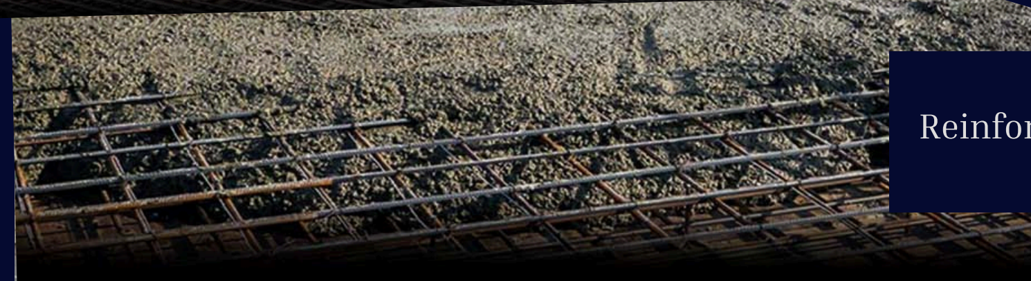
Reinforcement Of hollow block Slab
